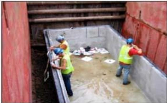
Left: 345 kV XLPE project – Cement vault visible with two chimneys extending up to be level with the future road surface.
